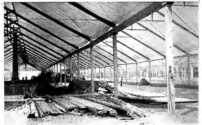
THE LARGE TENT AT THE "INTERNATIONAL" IN THE COURSE OF ERECTION.
